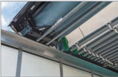
Hinteres Verdeckende · Rear end of roof
